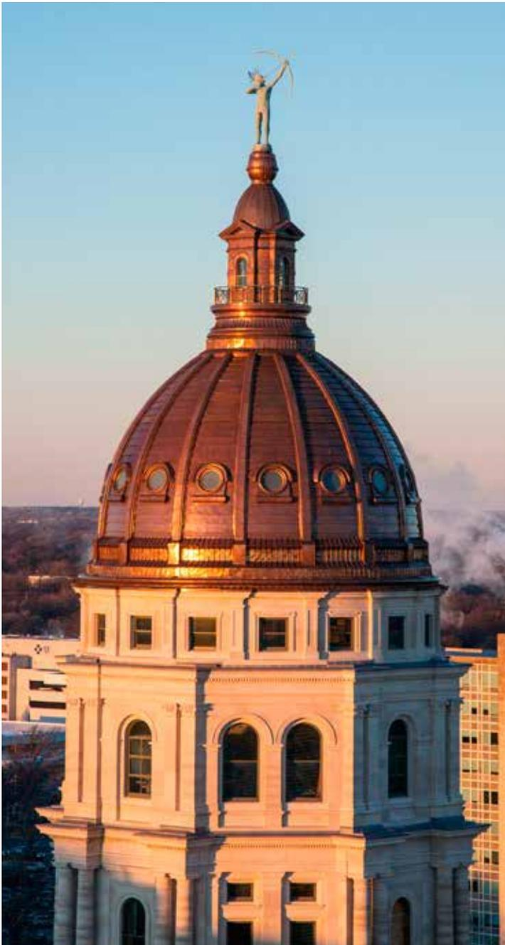
In addition to these panels, the dome incorporated new copper window surrounds, stainless steel gutter frames, heat trace, roof drains and lightning protection
