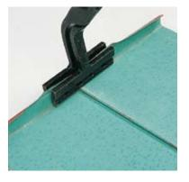
Use the seaming iron to erect the standing seam.
