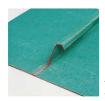
At the head end of the seam, 8–10 mm of the bead are flattened.
