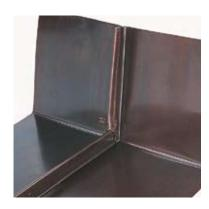
The abutment seam is repositioned and double-seamed.
