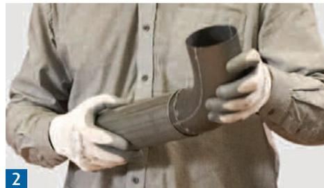
**2** Once measured, fit the two bends together. It may be necessary to extend the assembly using a piece of downpipe.
