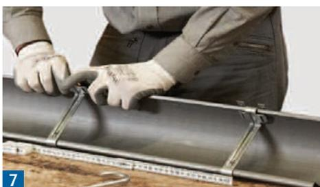
**7** Clip concealed brackets to the cut lengths of gutter at 400mm max centres.
