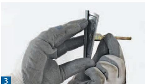
**3** At downpipe joints, mark positions for the v-locks at every 2 metres. Then firmly screw-fix the v-lock to the wall.
