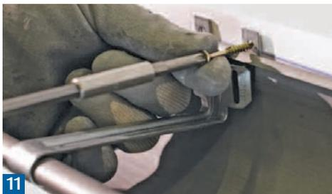
**11** Fix the gutter brackets according to the chalkline.
