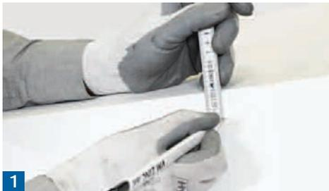
**1** Using a rule, make a chalkline setting the fall towards the running outlet and required position of the downpipe.
