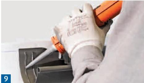
**9** Apply two, thin, parallel beads of VMZINC-G adhesive to the inner surface of the running outlet at max 50mm from the edge.
