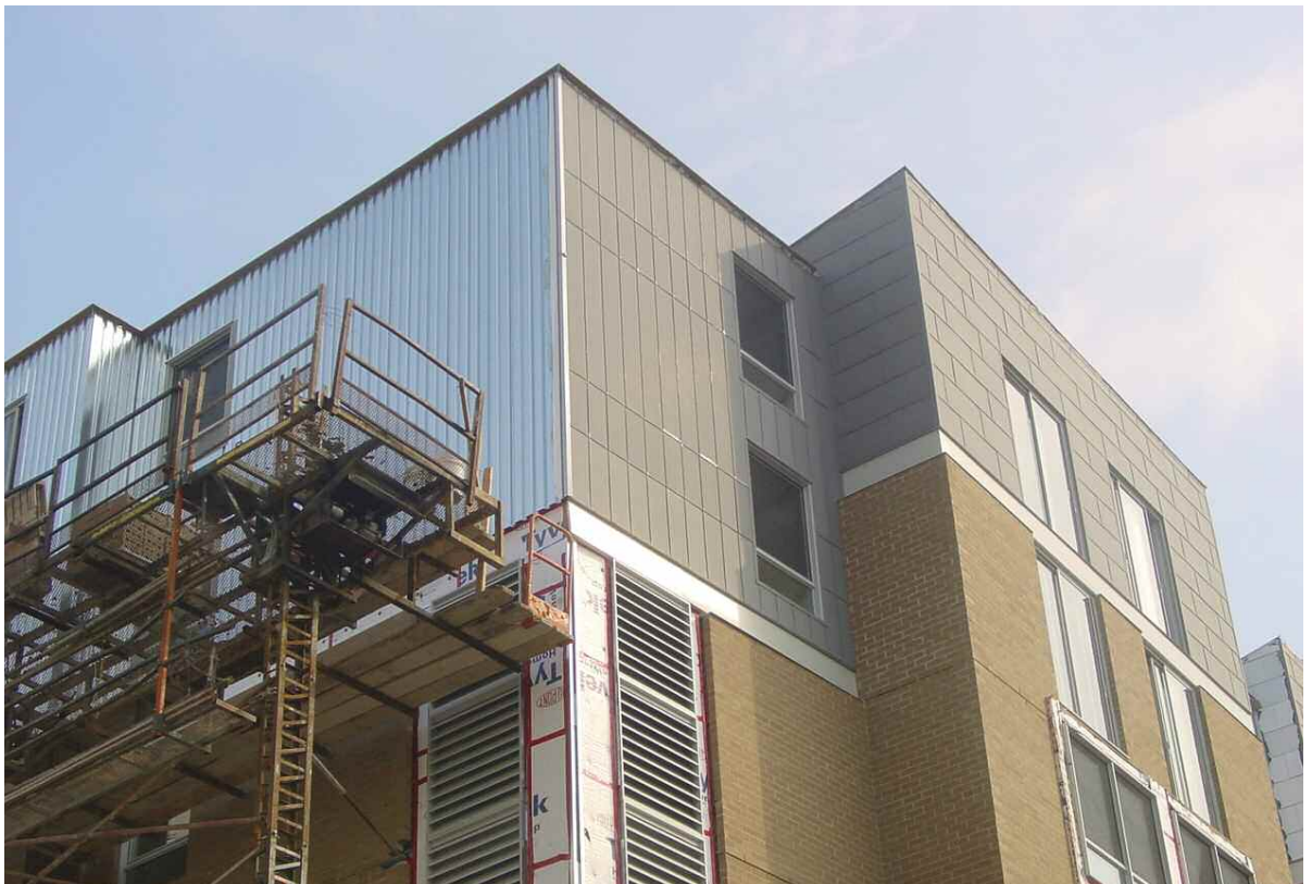
Example of galvanised steel deck being used as a substrate for flat lock wall panels
