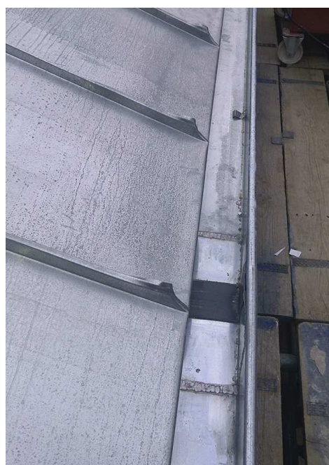
Expansion joint soldered to gutter
