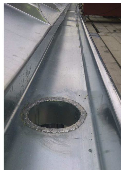
Downpipe outlet starter soldered to gutter
