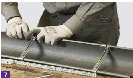
5 Firmly fix the prepared running outlet according to the chalkline.
